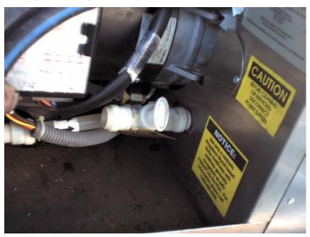
You will need to connect drain hose to the valve. In the example shown on the previous page, you would use either a short piece of pex pipe. Connect to a piece of clear 5/8" ID plastic pipe that is long enough to drain the coolant outside of your coach. In some coaches the valve may terminate in a  $\frac{1}{2}$ " NPT (standard pipe) threaded coupling.
