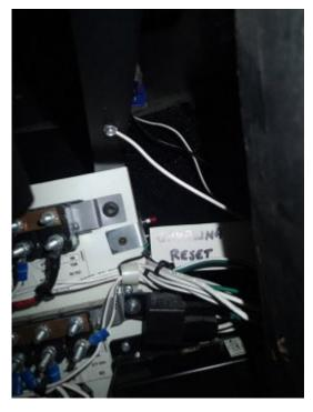
A picture of the reset switch I installed for the Javalina tank calibration. A big thanks to Mike O'Leary (previous owner who told me where to find the ground wire and to Barry Beam for pointing out that he has a push button switch on his system. The switch is in the upper right corner of the previous described panel.
