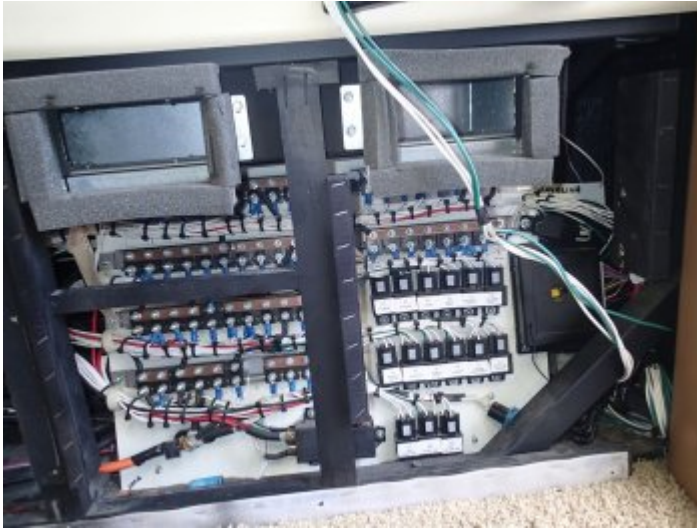
A picture of all the re-settable fuses behind this panel.
