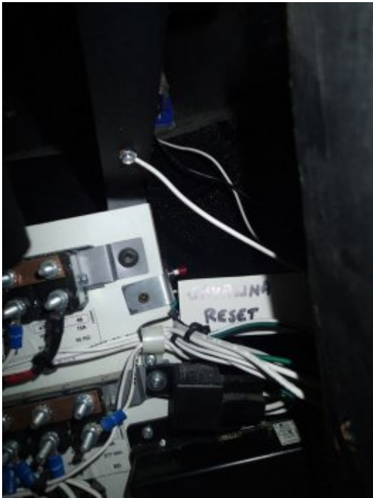
A picture of the reset switch I installed for the Javalina tank calibration. A big thanks to Mike O'Leary (previous owner who told me where to find the ground wire and to Barry Beam for pointing out that he has a push button switch on his system. The switch is in the upper right corner of the previous described panel.
