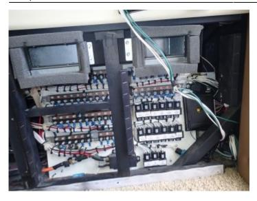
A picture of all the re-settable fuses behind this panel.
