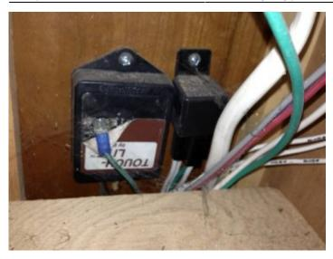
If you have problems with your porch light, the control box and relay are located inside (behind) the box next to the passenger seat, the one that holds a 110v plug, passenger side heater control, 12v outlet, slide cover switch and magazine rack. A new part and at least two hours labor (if you know where to look and know what you are doing) and you might be lucky to have 1/4 inch of wire to work with.
