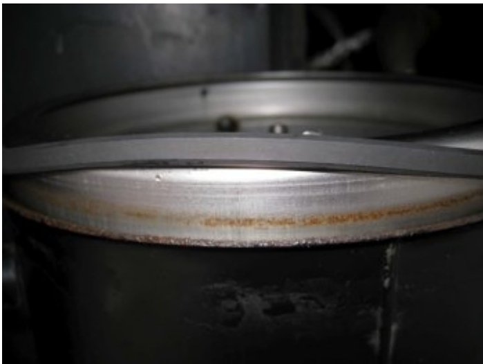
New gasket in place but not seated all the way down. When cover is placed on tank it seals against gasket forcing it
