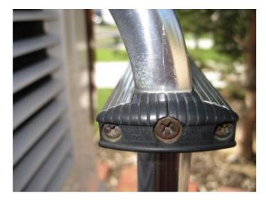
Cracked ends may be difficult to see. Crack usually happens in center.
