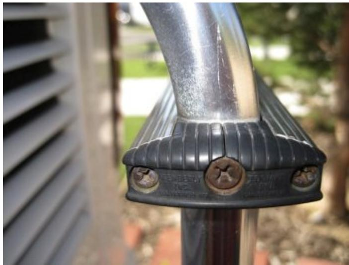
Cracked ends may be difficult to see. Crack usually happens in center.
